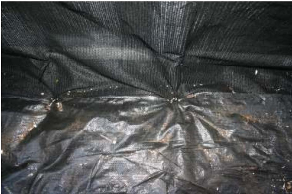
Plastic "weed mat" was used on the floor. It was attached to shade cloth lower edge using tent pegs.
