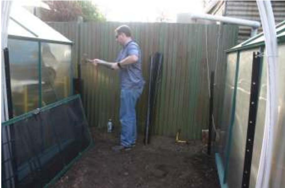
My son James banging in steel pickets for the anchor points of the frame. These could not be exactly lined up with the greenhouses as they have cement foundations at the corners, so the flight house is slightly set back.
