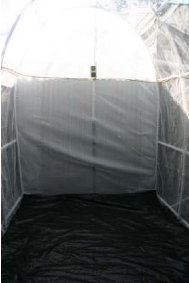
Rear wall from the inside showing misting tubes attached to the frame by cable ties.
